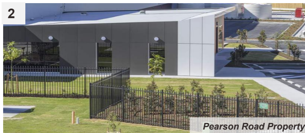
Drought resistant landscaping installed for water saving amenity
