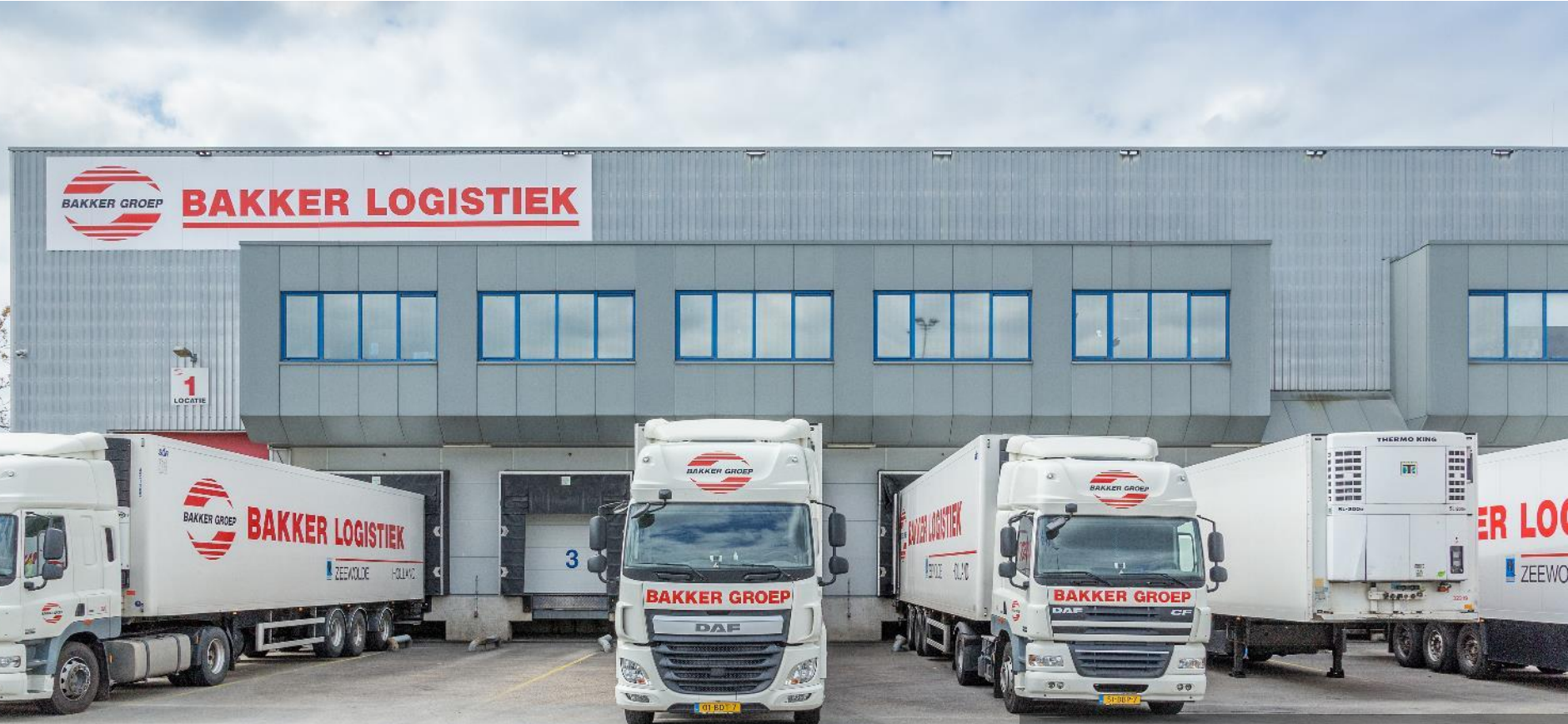
Bakker Logistics Facility, Zeewolde, The Netherlands
