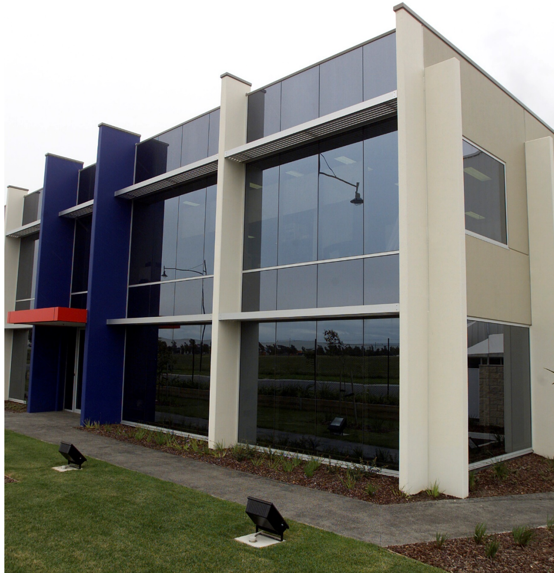
63-79 South Park Drive, Dandenong South, Victoria, Australia
