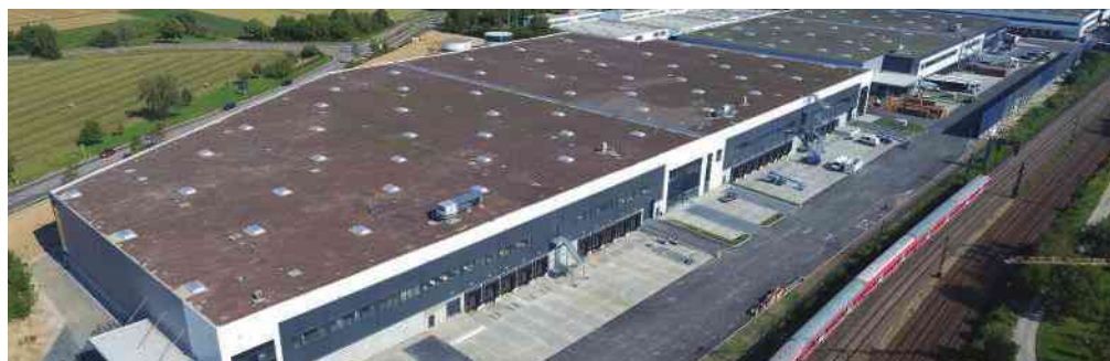
Bosch Facility, Germany
