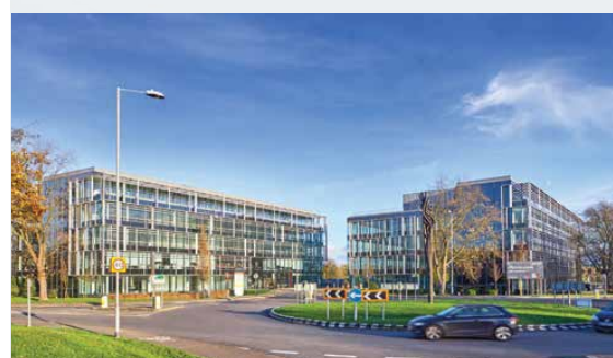
▲ Maxis Business Park, Bracknell, Thames Valley, the UK
