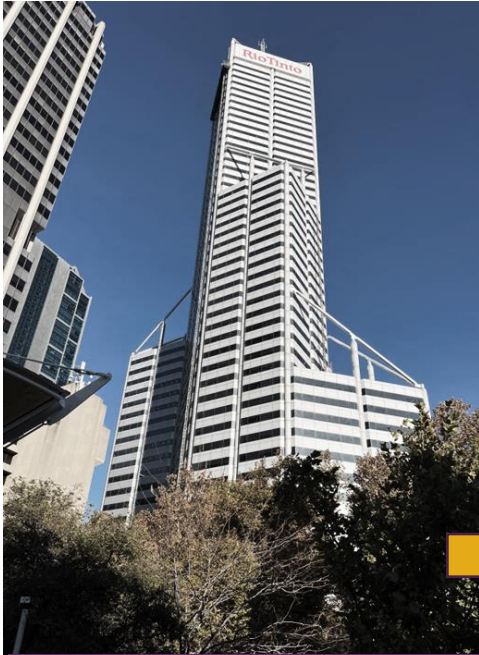
Before façade works
